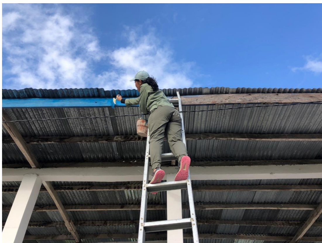
Repaint the tribune
